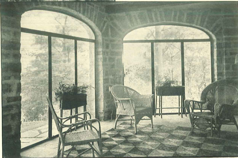
(Above)—This Higgin-screened out-door living room brings the joy of the surrounding woods into the room itself without annoyance of flies and other insects.
